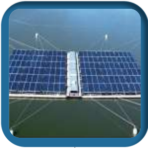
Mooring / anchoring device
