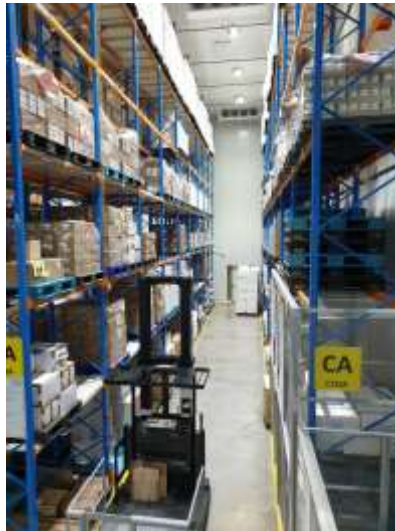
Cold Room, 2 to 8 deg C
