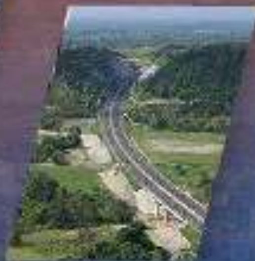
SUBIC-CLARK TARLAC EXPRESSWAY
